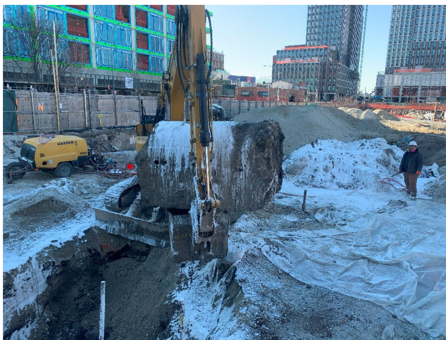
Photograph No. 10: Representative photo of Tank-11 removal on 3/01/24.
