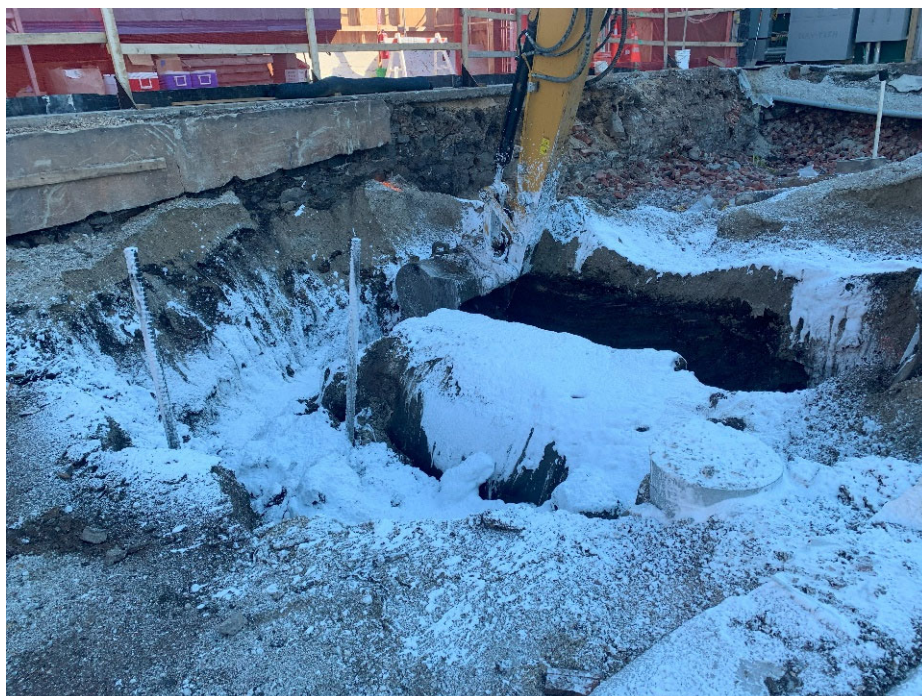
Photograph No. 9: Representative photo of Tank-11 removal on 3/01/24.
