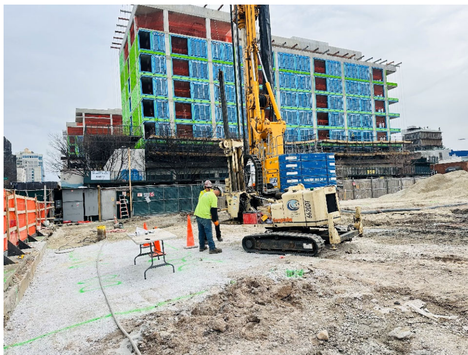
Photograph No. 19: Representative photo of delineation soil borings on 3/29/24.
