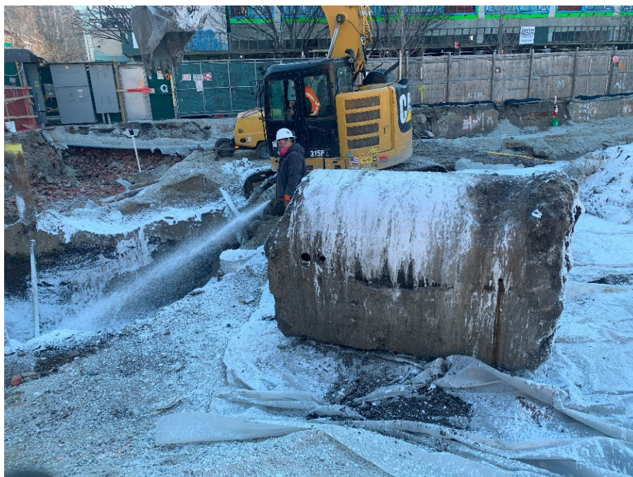
Photograph No. 13: Representative photo of Tank-11 on 3/01/24.
