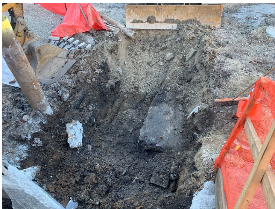
Photograph No. 2: Representative photo of Tank-11 located in grid O6, encased in concrete on 2/5/24.
