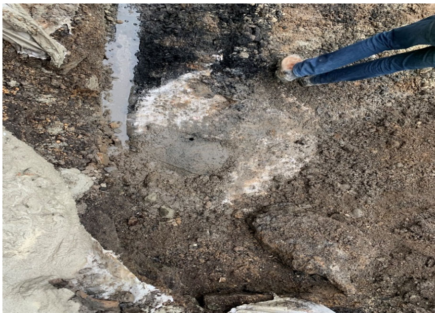
Photograph No. 1: Representative photo of Tank-11 located in grid O6, encased in concrete on 2/2/24.
