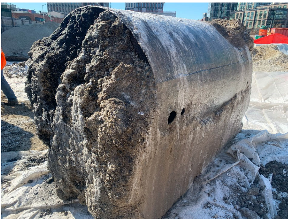
Photograph No. 11: Representative photo of Tank-11 on 3/01/24.
