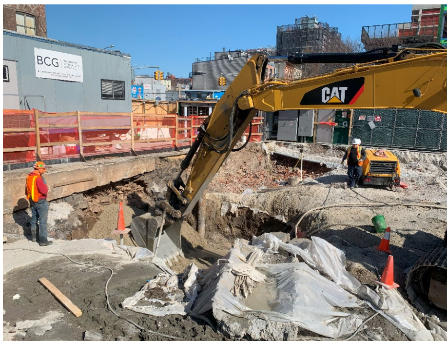
Photograph No. 16: Representative photo of temporary backfill placement on 3/12/24.
