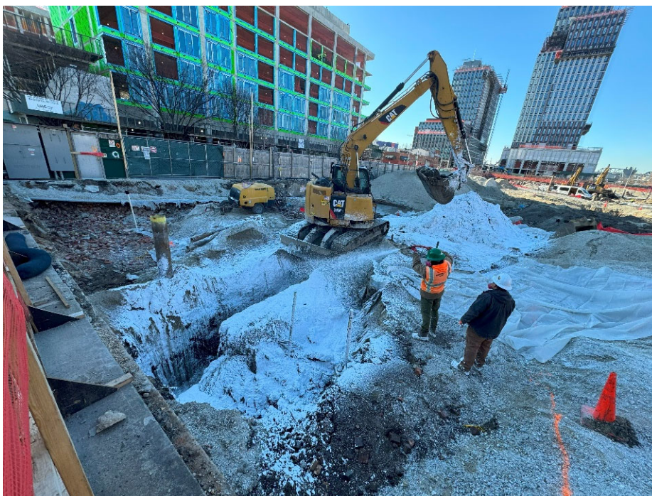
Photograph No. 12: Representative photo of excavation area and stockpile on 3/01/24
