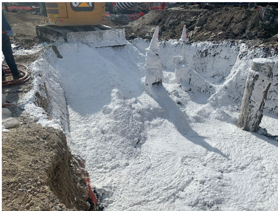
Photograph No. 18: Representative photo of additional excavation and ATMOS application on 3/13/24.
