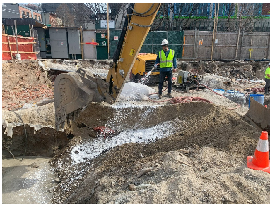
Photograph No. 17: Representative photo of additional excavation on 3/13/24.
