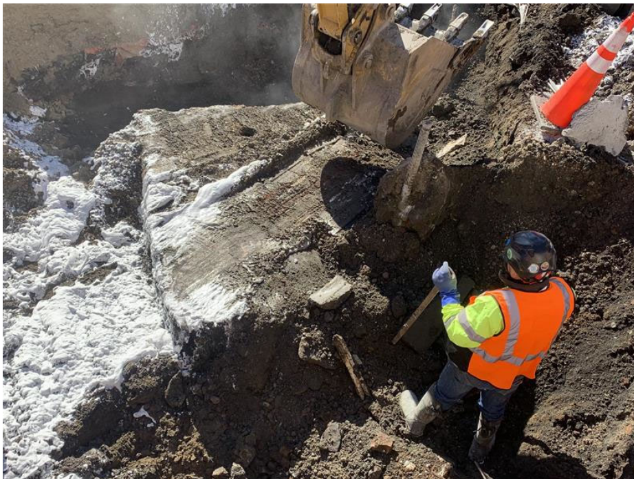
Photograph No. 6: Representative photo of tank located in grid O6, encased in concrete with ATMOS foam applied on 2/5/24.
