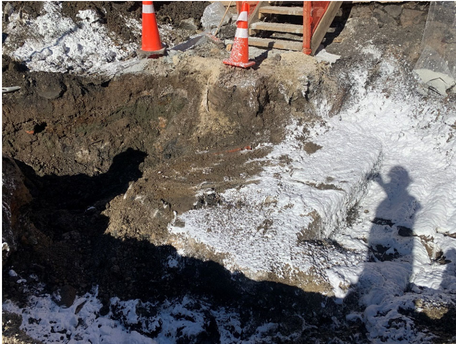
Photograph No. 5: Representative photo of tank located in grid O6, encased in concrete with ATMOS foam applied on 2/5/24.
