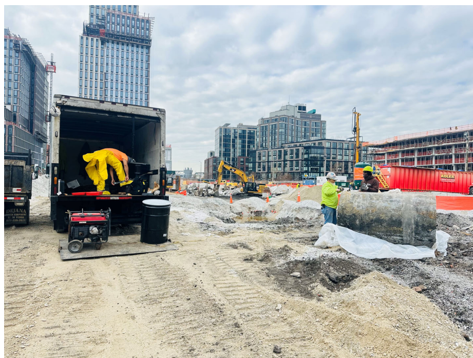
Photograph No. 14: Representative photo of PAL prepping Tank-11 for disposal on 3/04/24.
