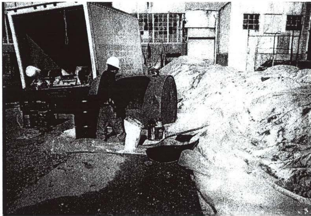
Photo 10 - No. 2 Fuel Oil UST: Petroleum Stained Soil in Area Being Removed
