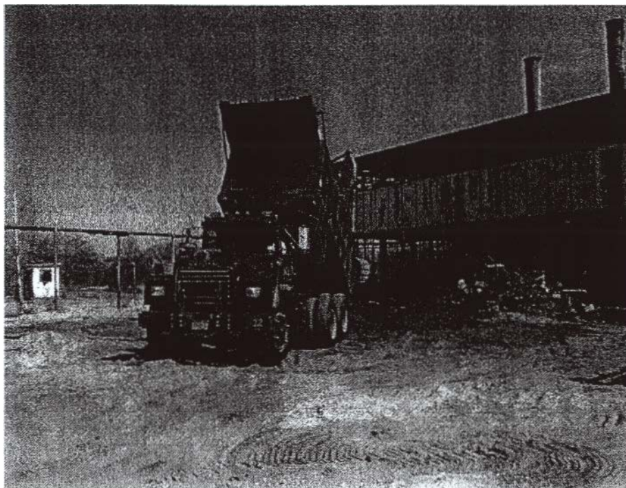
Photo 4 - Backfill Being Placed in Excavation
