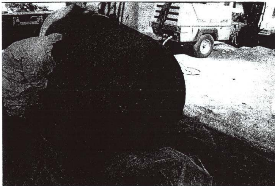
Photo 8 - Stained Soil Above No. 2 Fuel Oil UST in Area of Fill Pipe
