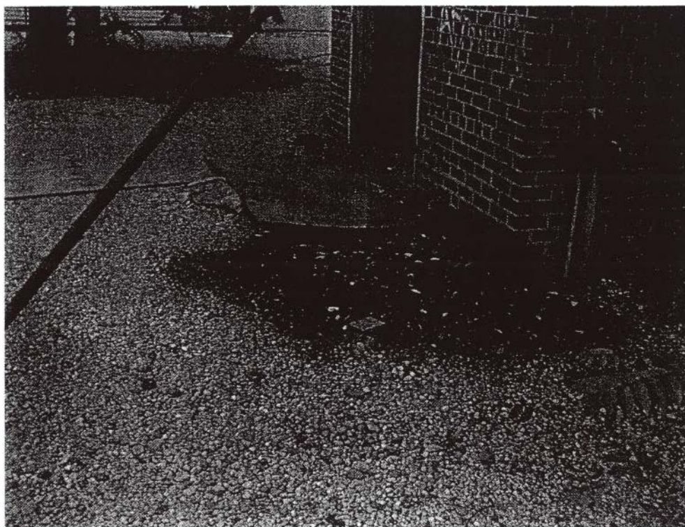
Photo 8 - Stained Soil Above No. 2 Fuel Oil UST in Area of Fill Pipe
