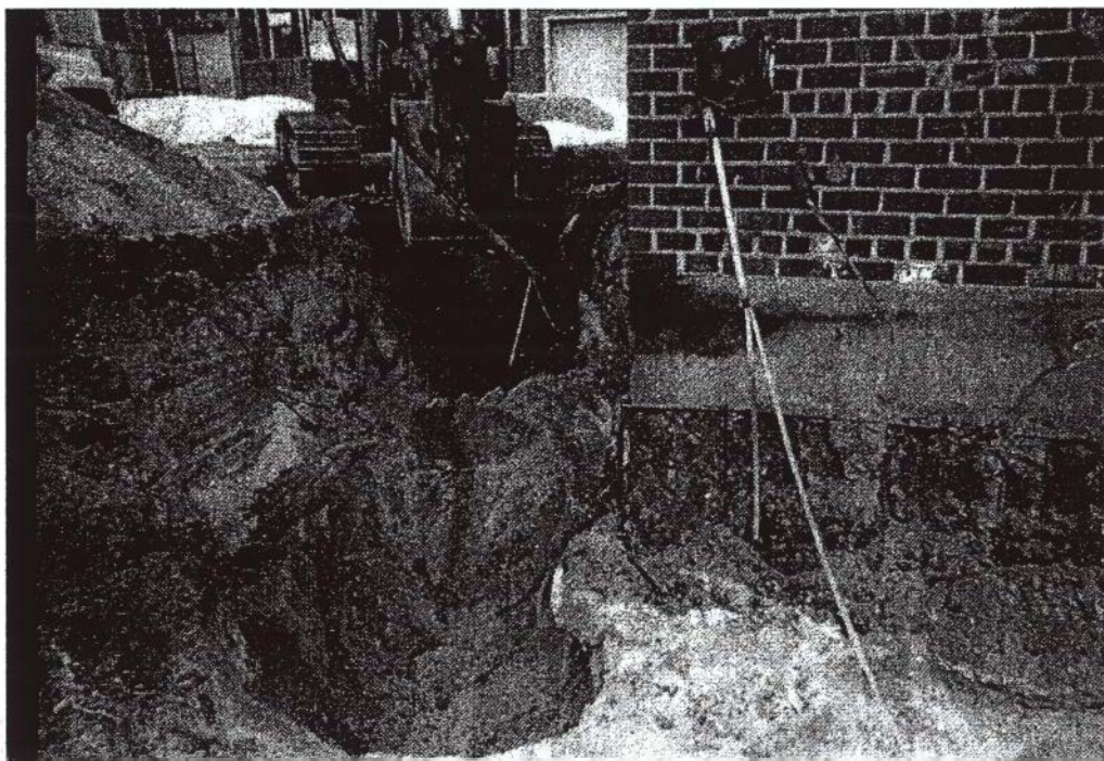
Photo 10 - No. 2 Fuel Oil UST: Petroleum Stained Soil in Area Being Removed
