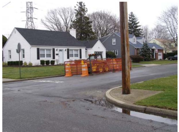
VP-116/MW116-5 Site After MR Rig Demobilization (Pending Development)
