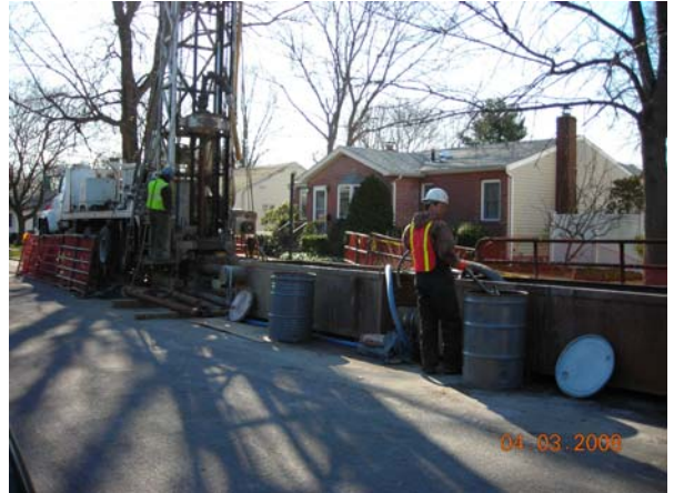
VP-113 Drilling Looking East
