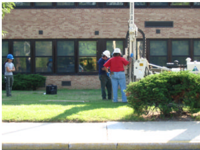
Installation of Soil Vapor Point
