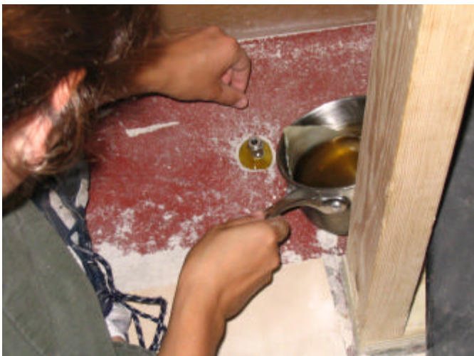
Sealing Sub-Slab Sample Point with Melted Beeswax
