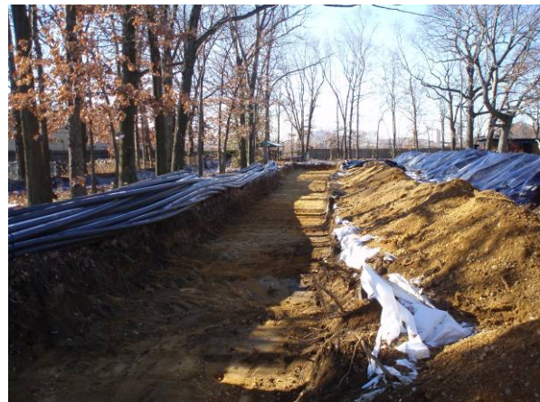
Trenching in McKay Field
