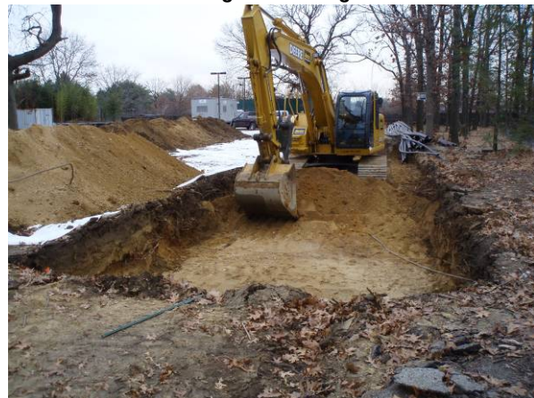
Trenching in McKay Field
