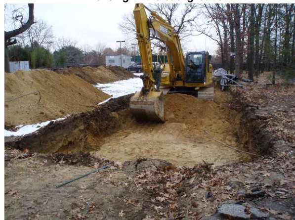
Trenching in McKay Field
