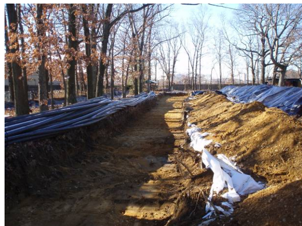
Trenching in McKay Field
