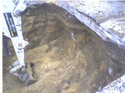
Trenching Along Southern Access Road
