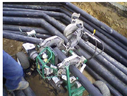
Fusing of Piping at Turn in Trench
