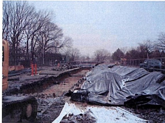
Trench Along Western Leg
