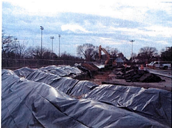
Trench Along Western Leg
