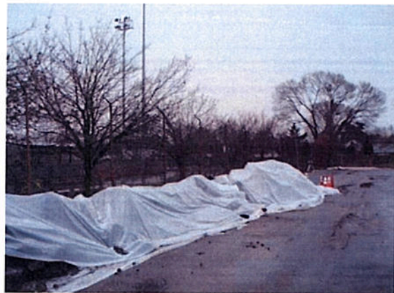
Staged Asphalt Along Western Leg
