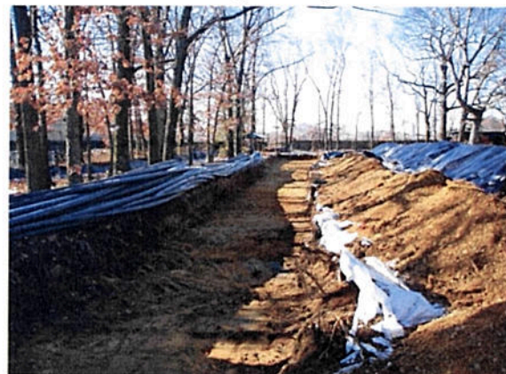
Trenching in McKay Field
