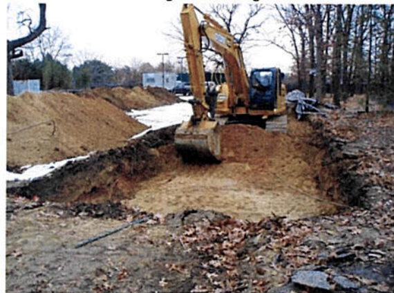
Trenching in McKay Field
