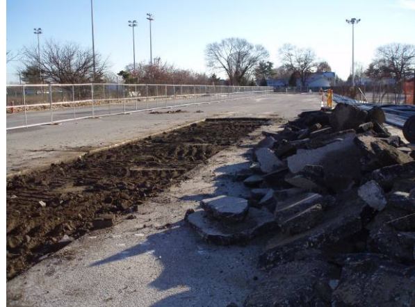
Asphalt Removal on Western Leg with Construction fencing in the background.
