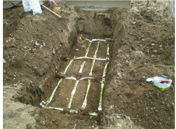
Warning Tape within Trench
