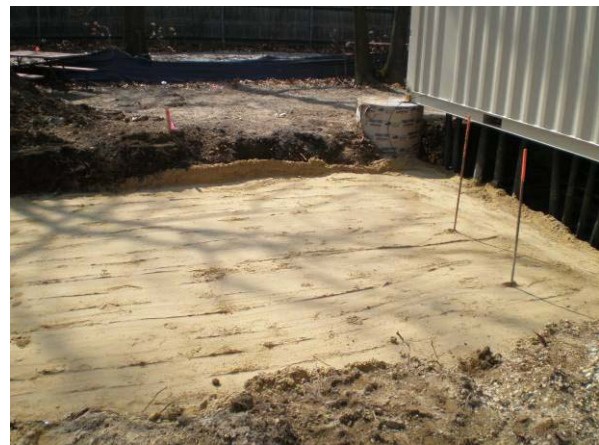
Backfilling in McKay Field
