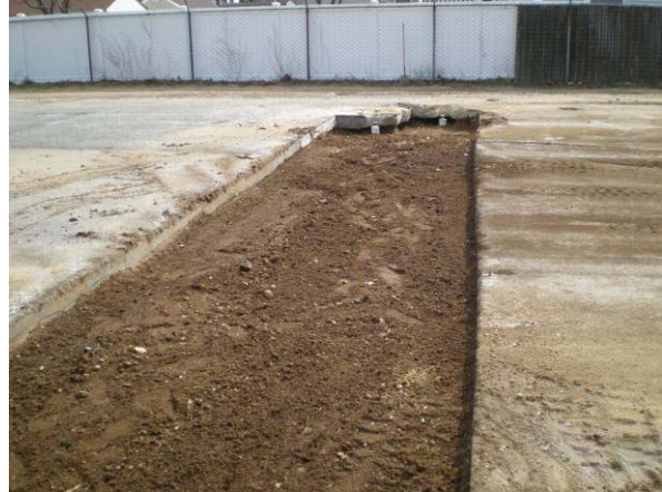
Backfill on Southern Access Road
