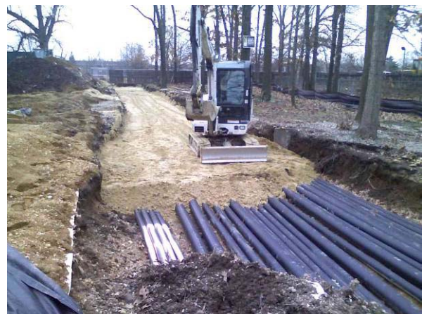
Backfilling in McKay field
