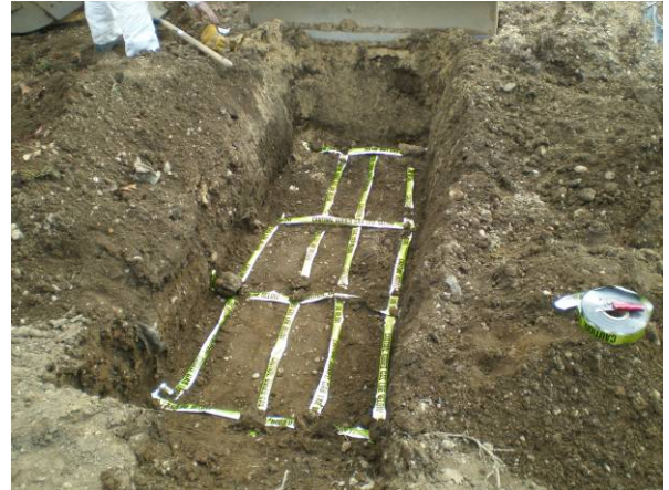
Warning Tape within Trench
