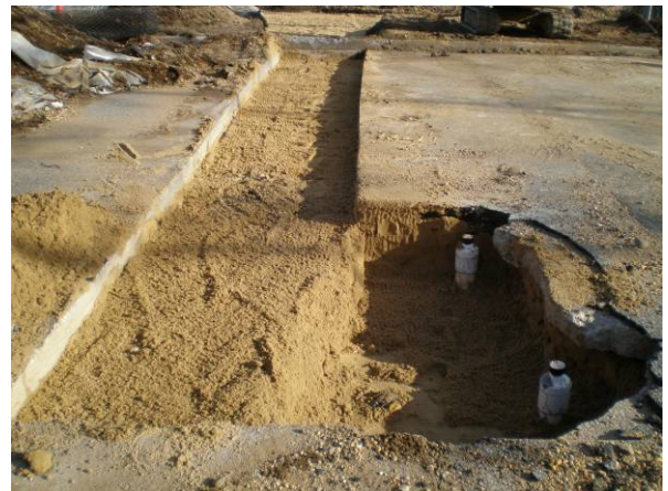
Western Leg Trenching to Wells
