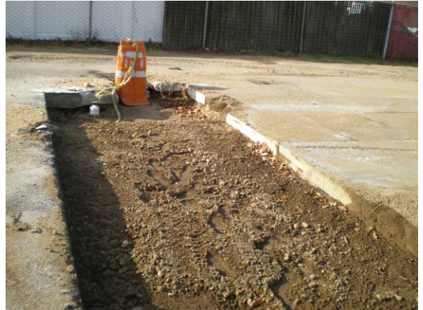
Trenching to Wells
