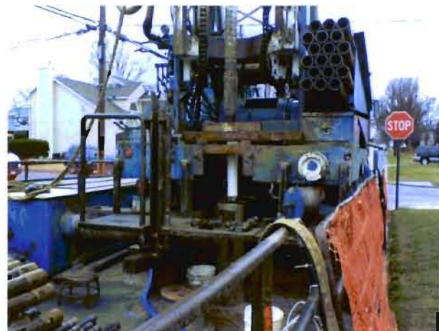
Well MW116-5 Installation (white PVC pipe)
