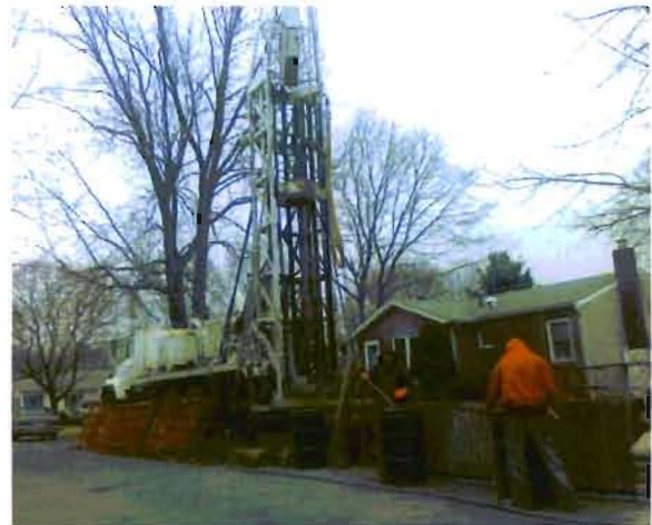
VP-113 Drilling Looking East
