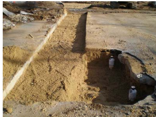
Western Leg Trenching to Wells
