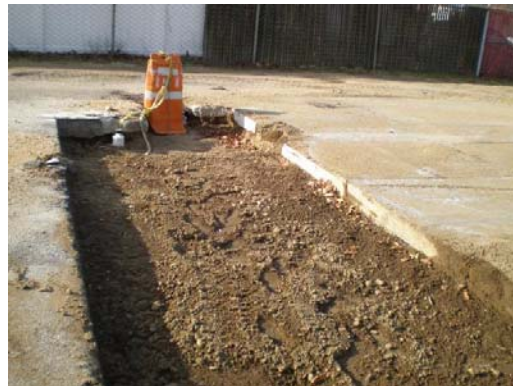
Trenching to Wells
