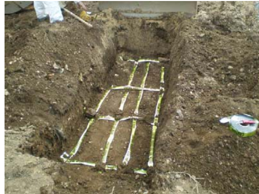
Warning Tape within Trench
