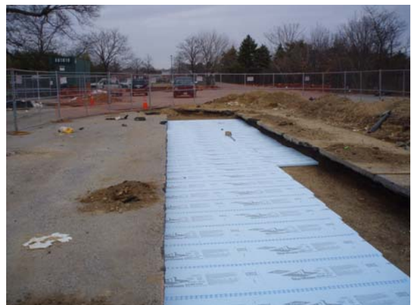
Installation of Insulation
