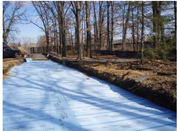
Installation of Insulation
