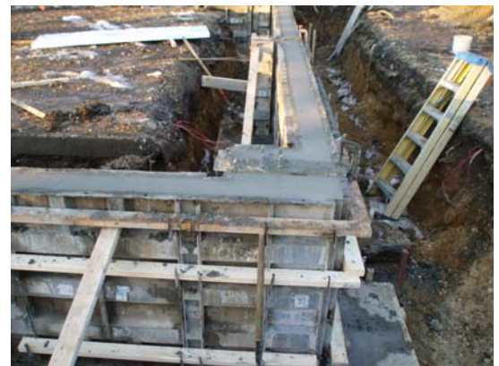
Treatment Building Grade Beams Poured with Southeast Anchor Bolts Showing
