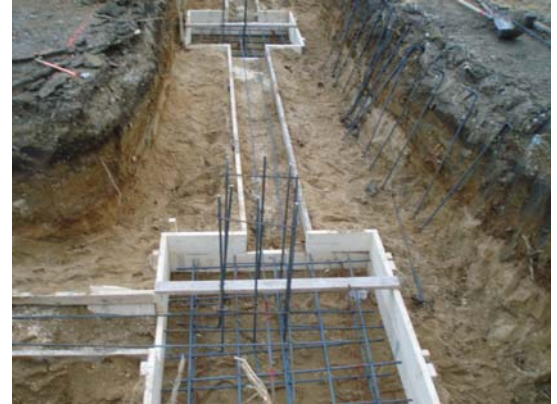
Forms and Rebar Installed for Treatment Building Footers and Grade Beams
