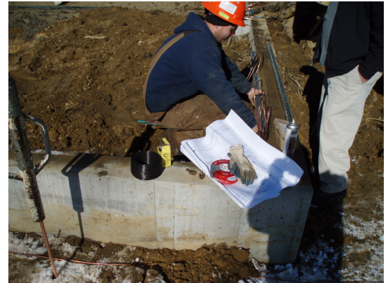
Treatment Building Grounding Grid Being Installed
