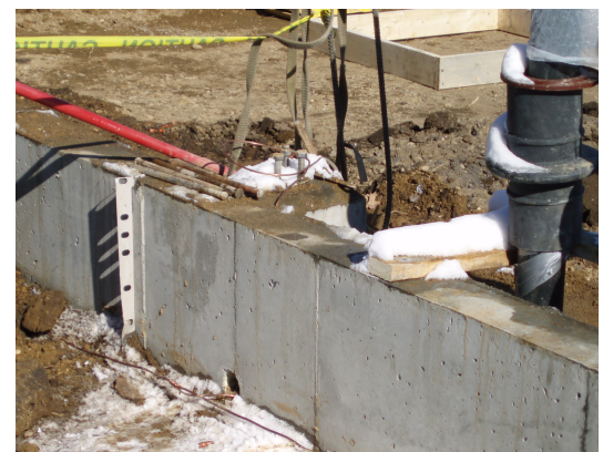
Backfilled Grade Beam and Pipe Sleeve for Influent Line
