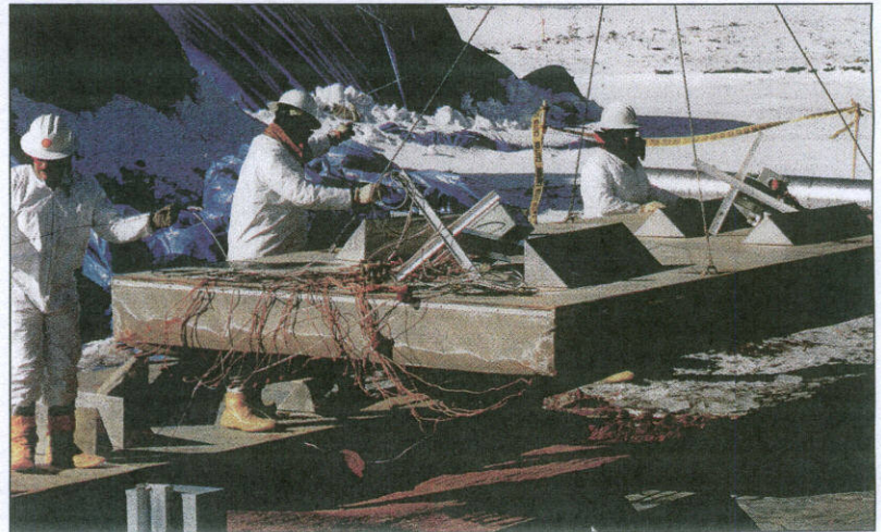
Thermal Blanket being lowered into position
