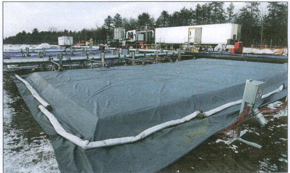
Thermal Blankets in place and operating
