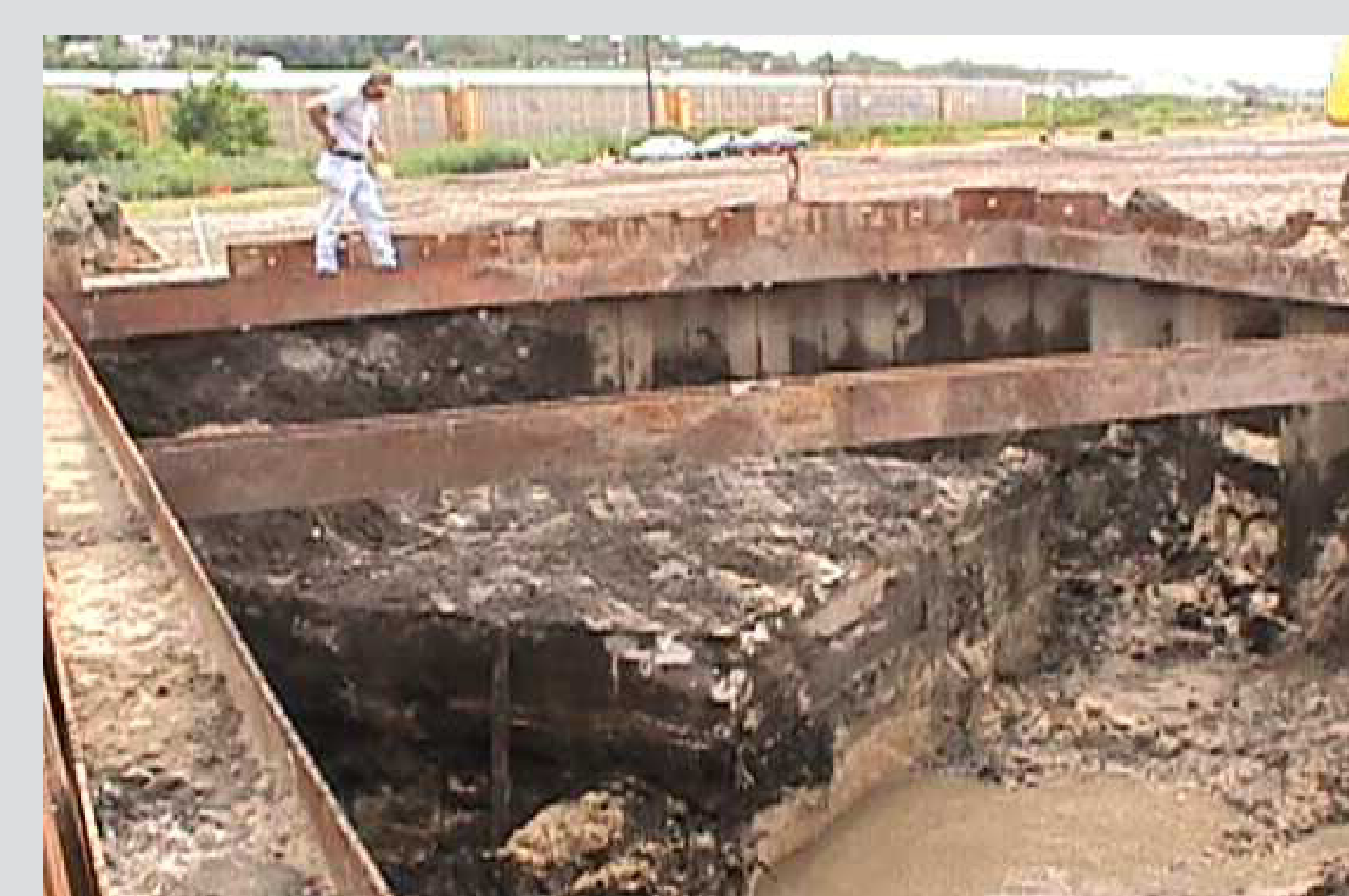
July 2006: B-5 Area Soil Excavation (after which soil was placed within one of the thermal treatment zones).
