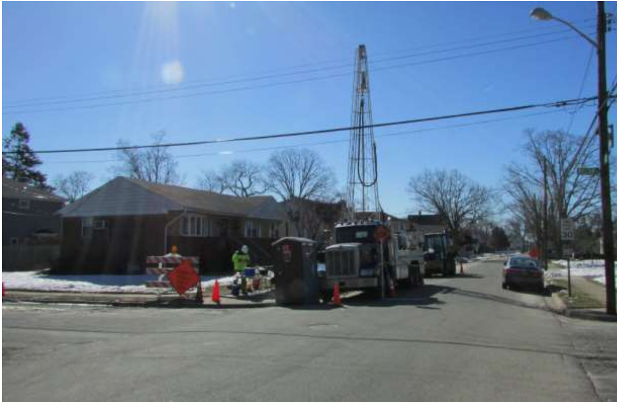
Intersection William and Broadway Streets, borehole drilling Northrop-Grumman 3/12/2015
