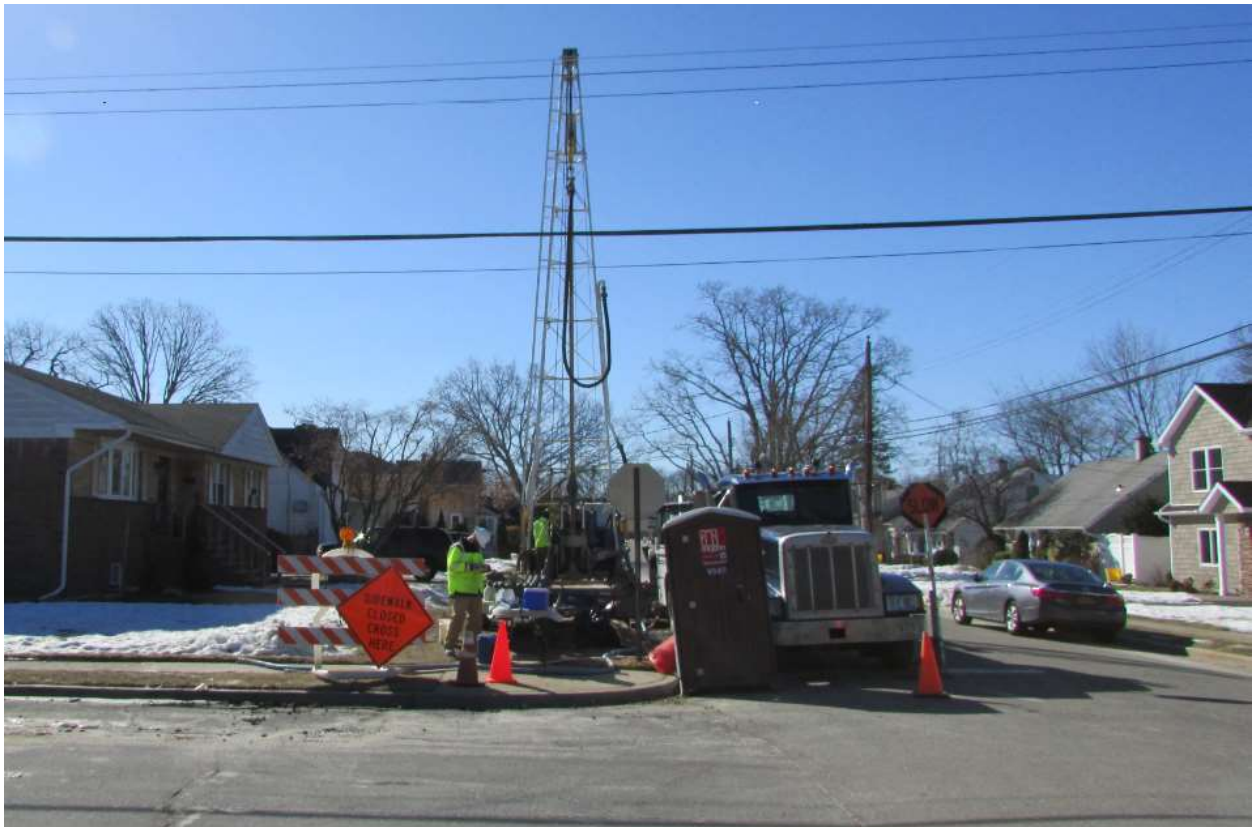
Intersection William and Broadway Streets, borehole drilling Northrop-Grumman 3/12/2015
