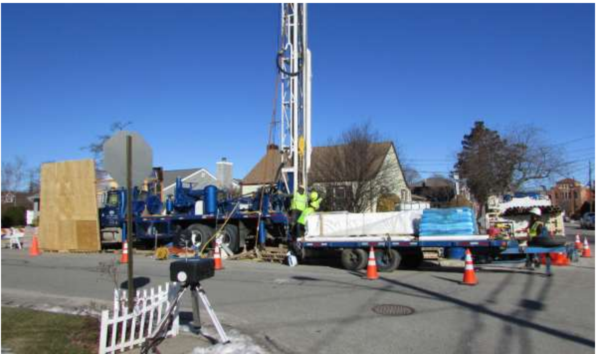
Intersection Emma and Windhorst Streets; Monitoring Well Installation Northrop-Grumman 3/12/15
