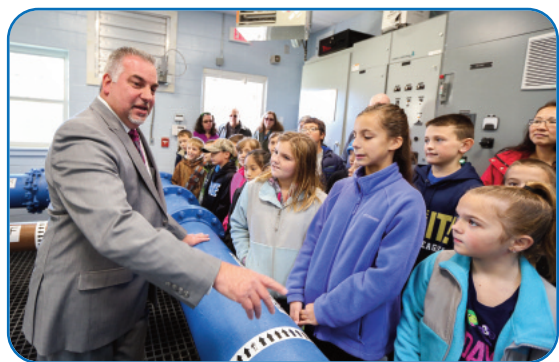
Superintendent Michael Boufis guided students around the pump station, explaining how it functions and provides the highest quality of water possible to the community each day.
