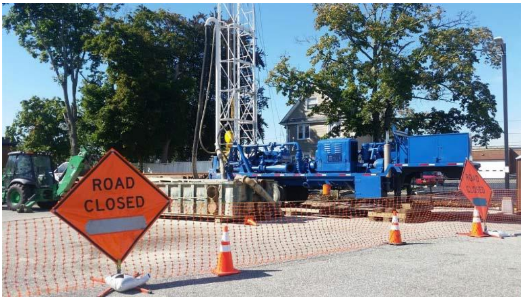
Typical Drilling of Extraction Well
