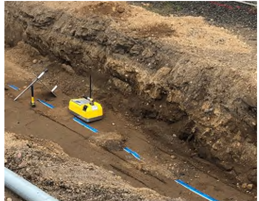
Density testing adjacent to HDPE piping
