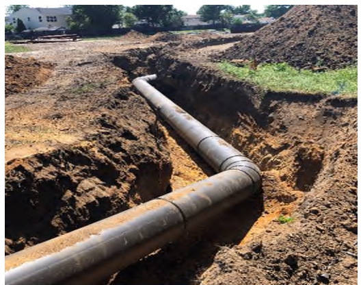
Partially installed 45-degree HDPE pipe section
