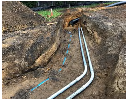
Communication conduits and HDPE pipe marking tape
