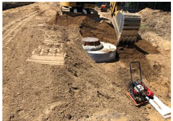
Placing backfill around leak detection vault near Station 6+00
