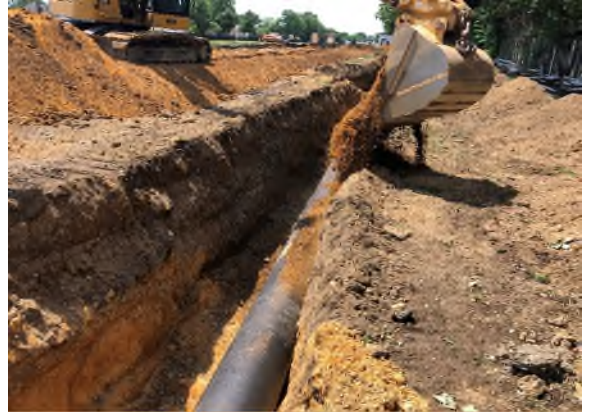
Placing backfill near Station 7+00
