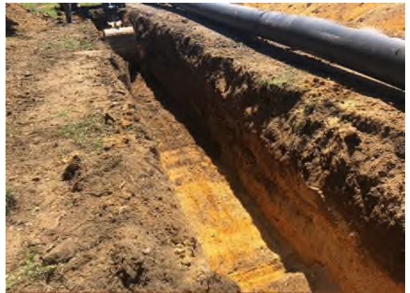
Excavating soil near Station 6+50
