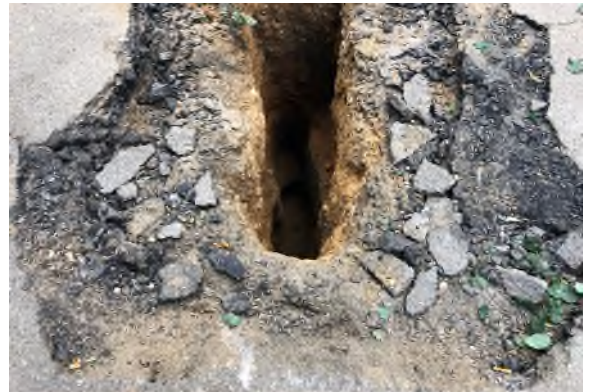
Vacuum excavating for utility location
