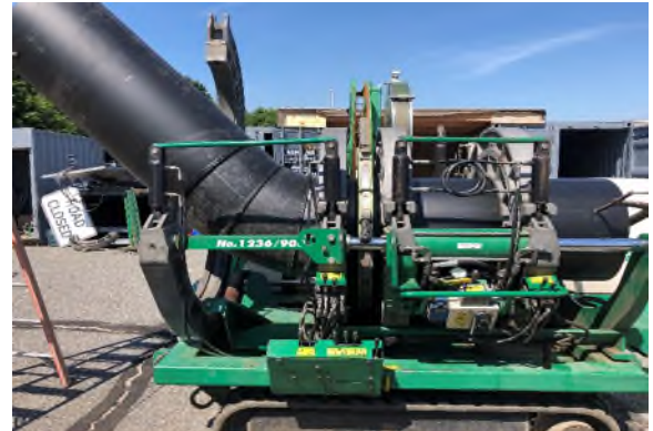
Construction of 122-degree HDPE pipe radius
