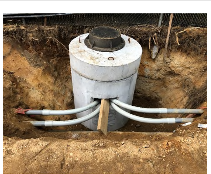
Leak detection manhole vault, lid, and cover at Station 0+48 in the Corridor
