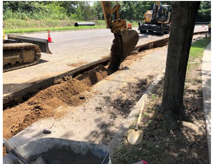
Placing backfill
