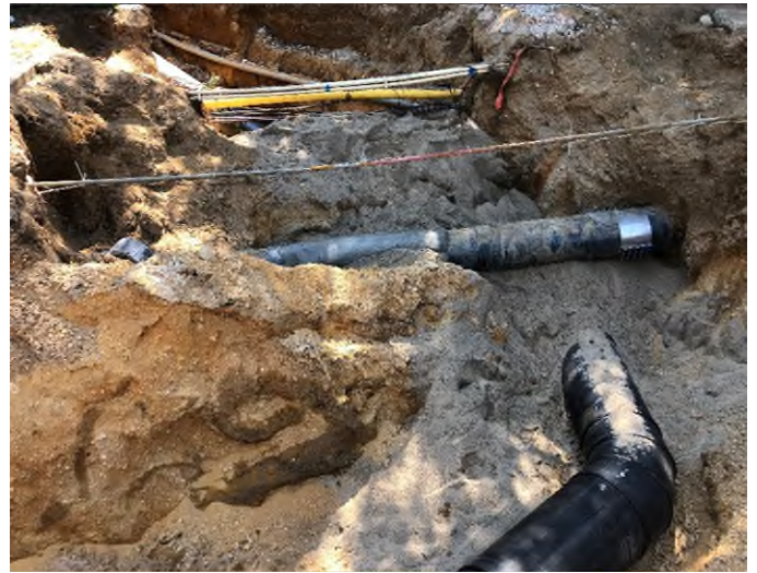
Utilities at the 122-degree HDPE pipe radius
