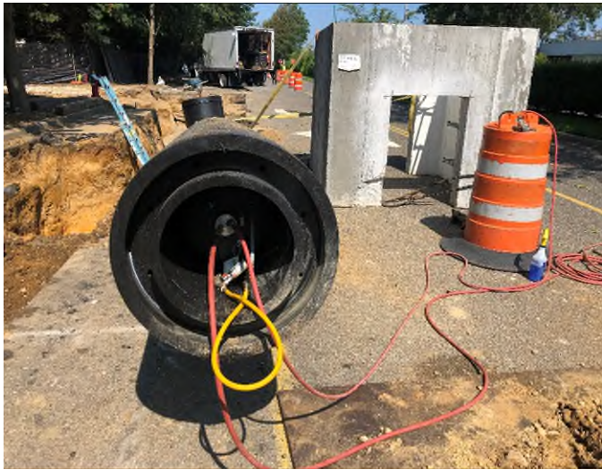
Pressure testing 16-inch HDPE carrier piping
