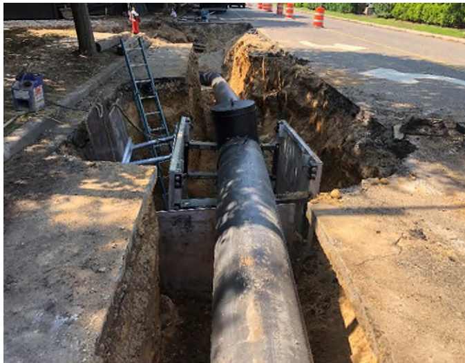
HDPE piping staged in the trench pending additional fusing and backfill
