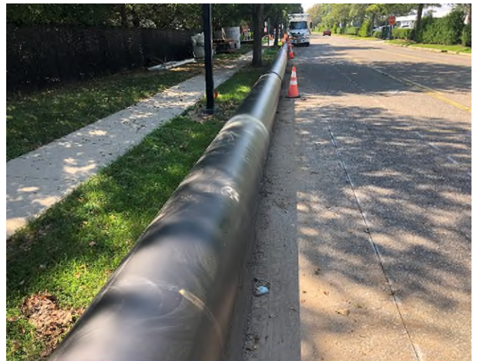
Fused HDPE piping staged along Grumman Road East pending installation
