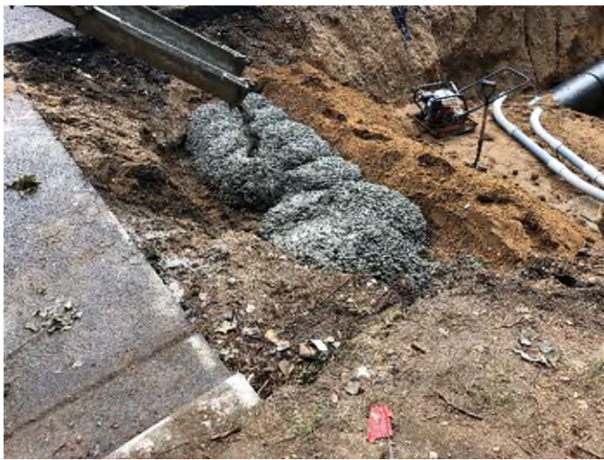
Placing concrete above the electric lines crossing Grumman Road East
