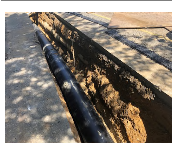
HDPE pipe under storm sewer lines near Station 8+00
