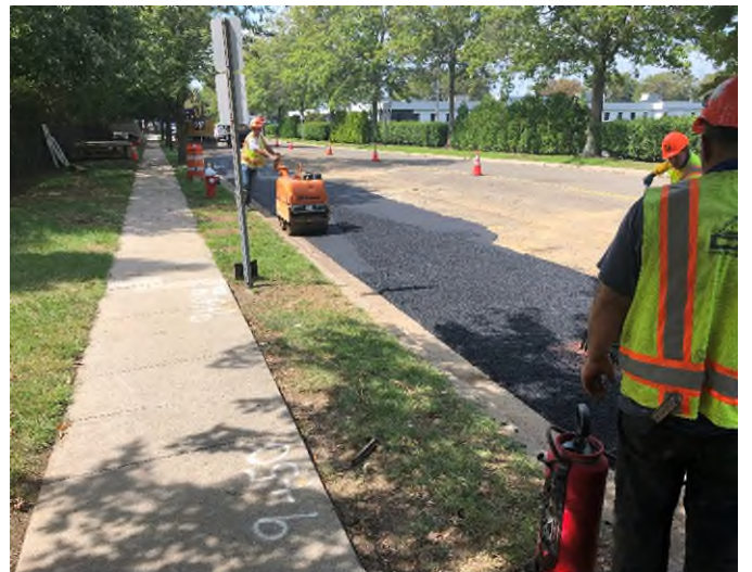
Compacting asphalt binder
