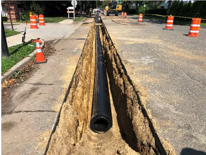
HDPE piping from Station 12+48 toward Station 14+00 along Grumman Road East
