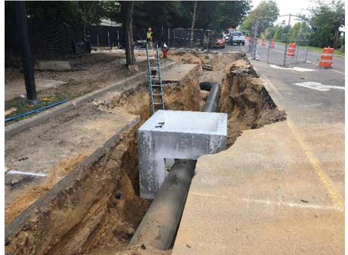
Air release vault riser at Station 13+78 along Grumman Road East
