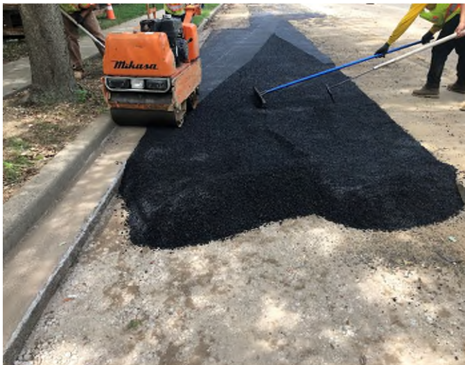
Placing asphalt binder
