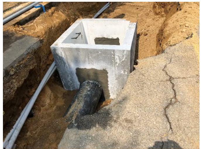
Air release vault riser with opening grouted at Station 13+78 along Grumman Road East
