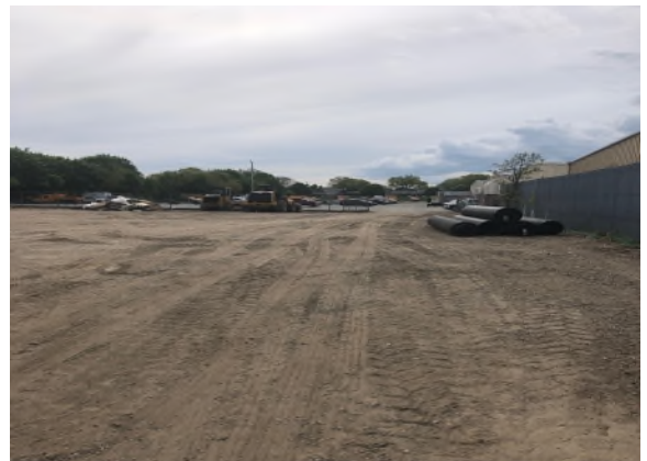
Pavement Removed from North Side of Building Site
