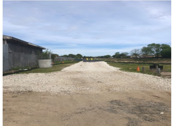
West End of Paved Access Road Along Basins
