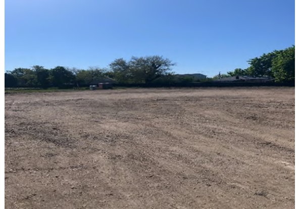
Pavement Removed from Construction Area
