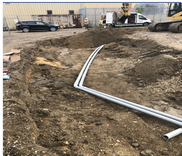
Backfilling Leak Detection Conduits
