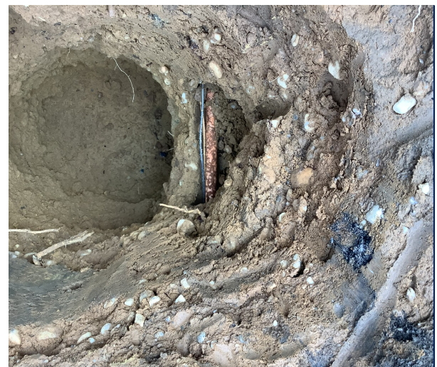
Located Plastic Gas Line with Tracer Wire at Sta. 19+60
