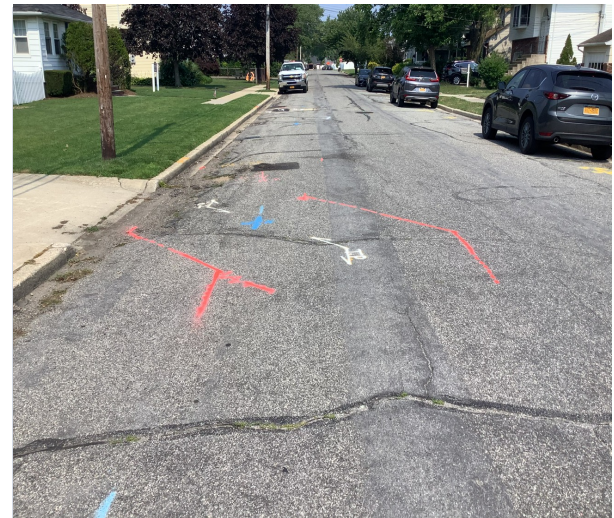
Trench Line Mark-out near Sta. 34+00
