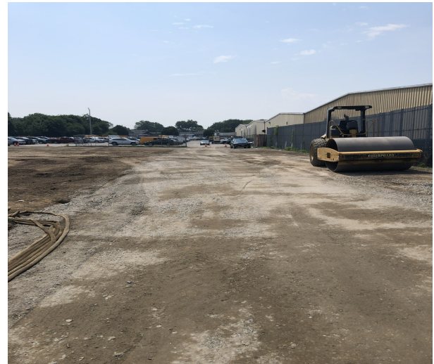
Backfilled Influent Pipeline
