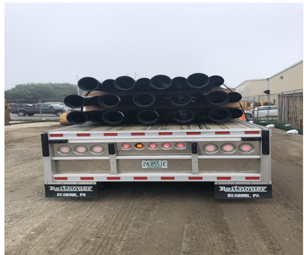
Delivery of Potable Water Pipe
