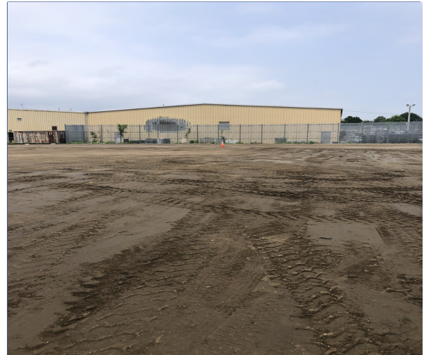
Backfilled Influent and Effluent Pipe Trenches
