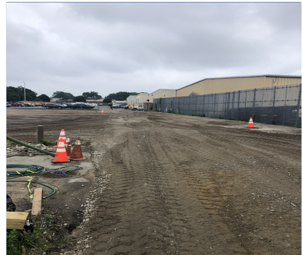
Backfilled Influent Pipe Trench
