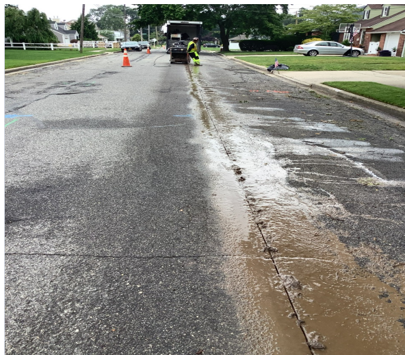
Saw Cutting Pavement on N Herman Ave
