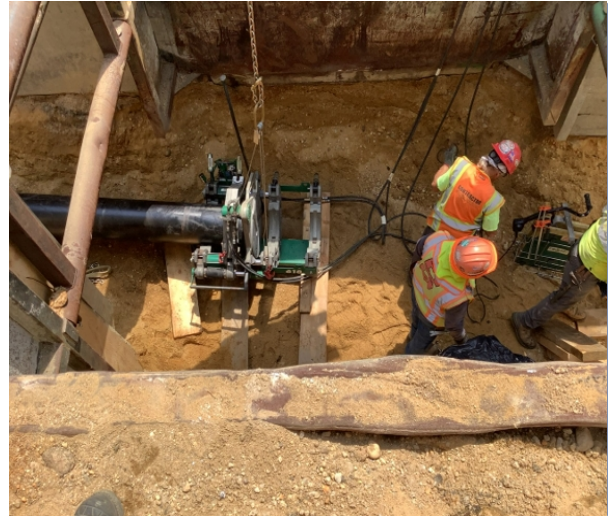
Fusing HDPE Pipe
