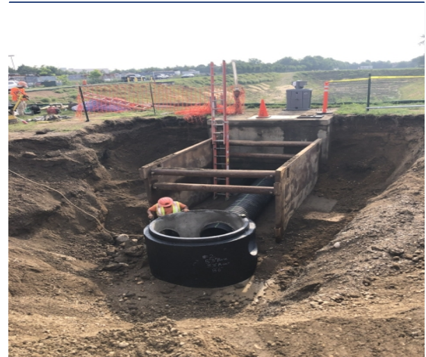
Storm Sewer Manhole MH-2 and Control Chamber A
