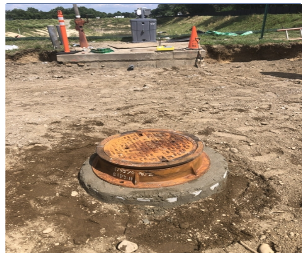
Top of Storm Sewer Manhole MH-2
