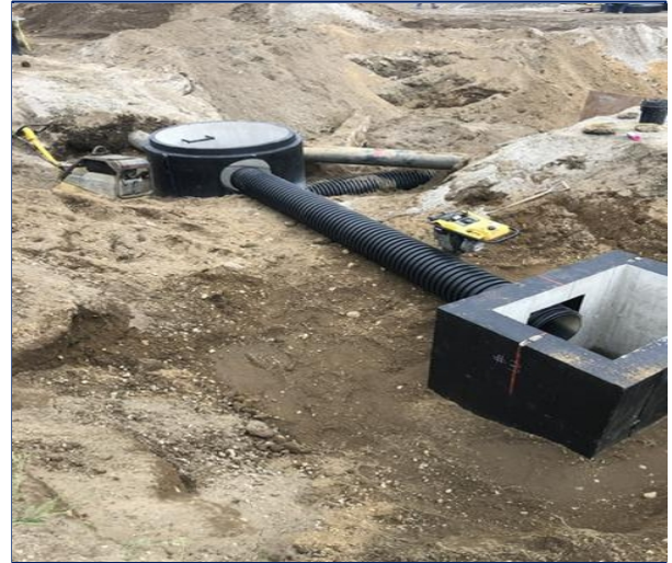
Storm Sewer Manhole MH-1 and Catch Basin CB-3
