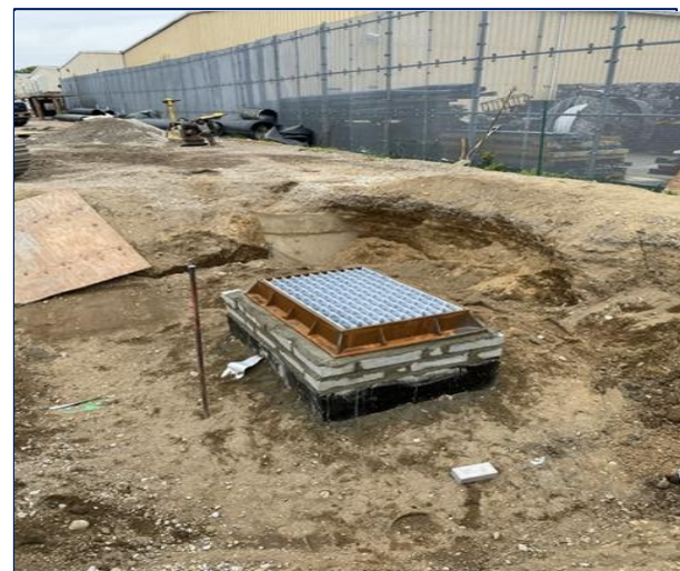
Top of Storm Sewer Catch Basin CB-2
