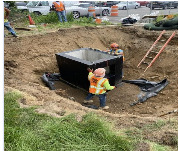
Installing Storm Sewer Catch Basin CB-4
