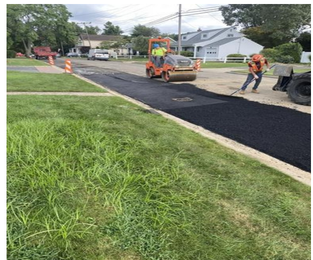
Placing Asphalt on N Herman Ave
