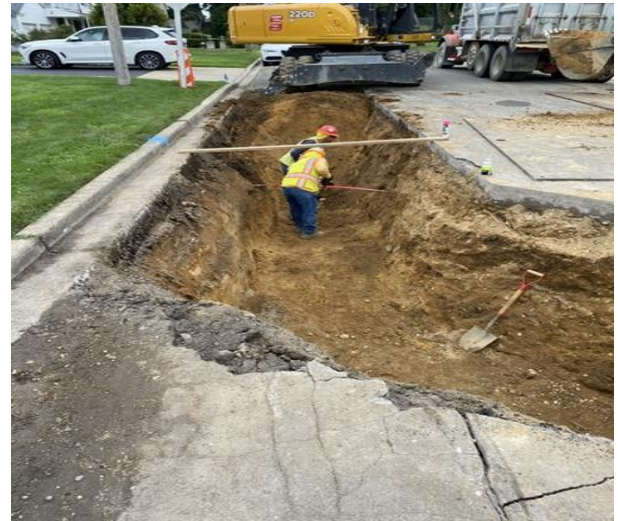
HDPE Pipe Trench on N Herman Ave
