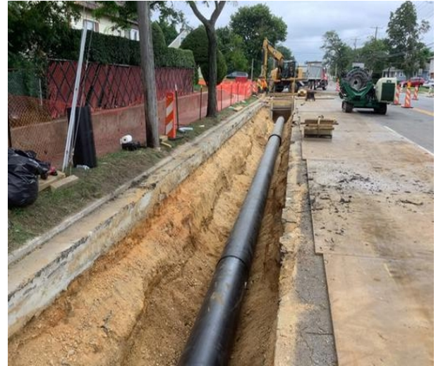
Installing HDPE Pipe on Stewart Ave
