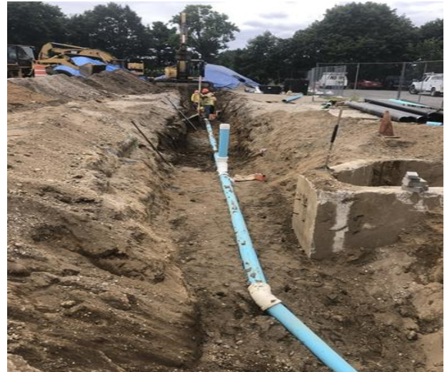
Installing Sanitary Sewer Piping
