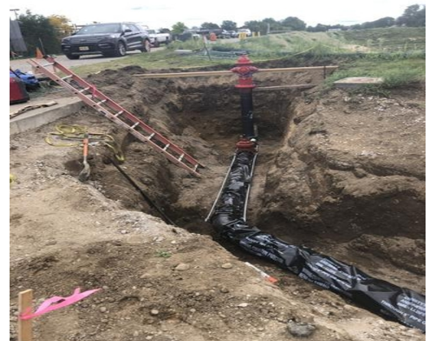
Installing Hydrant and Fire Protection Piping
