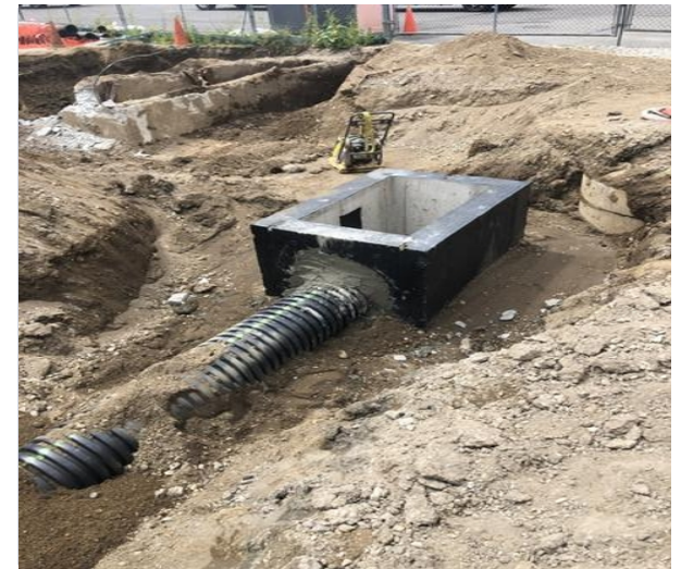
Installing Storm Sewer Catch Basin CB-1
