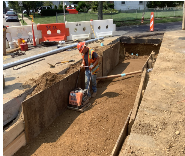
Backfilling and Compacting Trench on Stewart Ave
