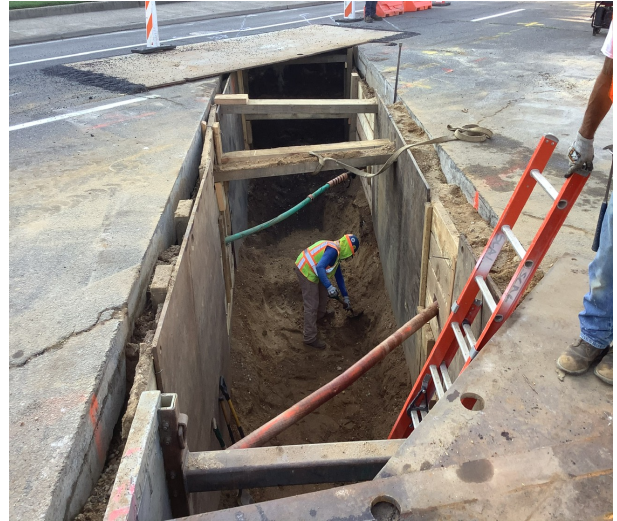
Excavating and Shoring Trench on Stewart Ave
