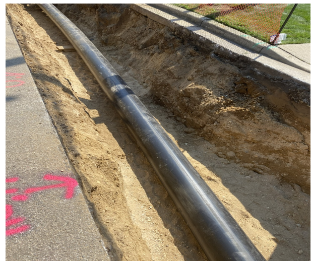
Installing HDPE Piping on N Herman Ave
