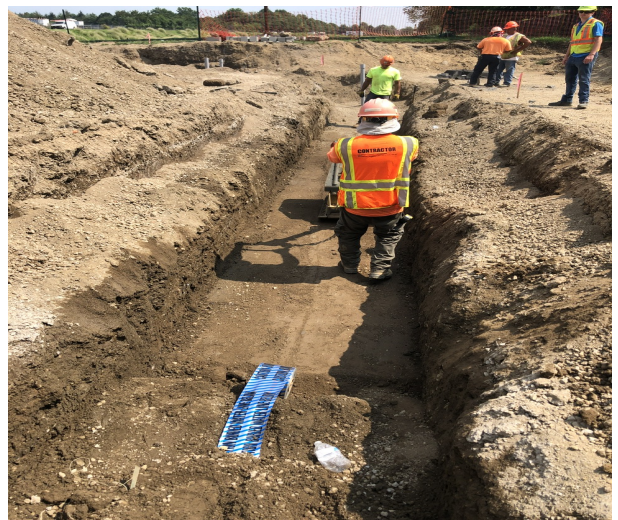
Backfilling Fire Protection Piping Trench
