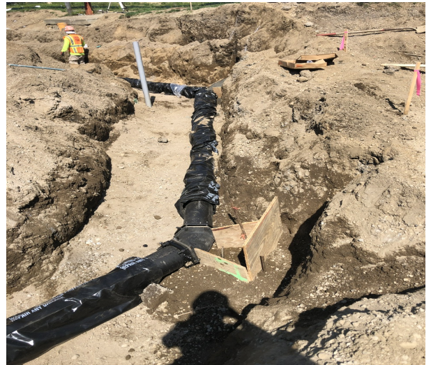
Installing Fire Protection Piping
