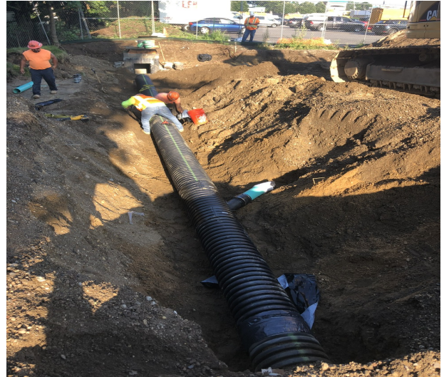
Installing Storm Sewer Piping to Catch Basin CB-4
