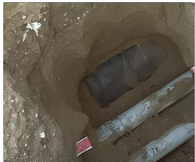
Locating Previously Installed HDPE Pipe on Seaman Ave
