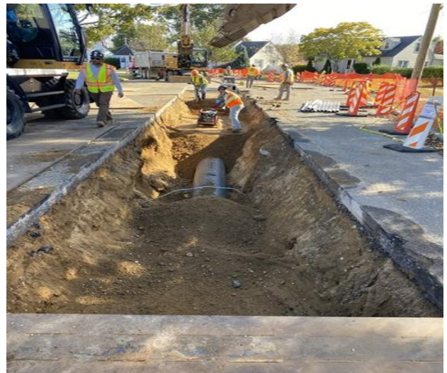
Backfilling Pipe Trench on S Pershing Ave
