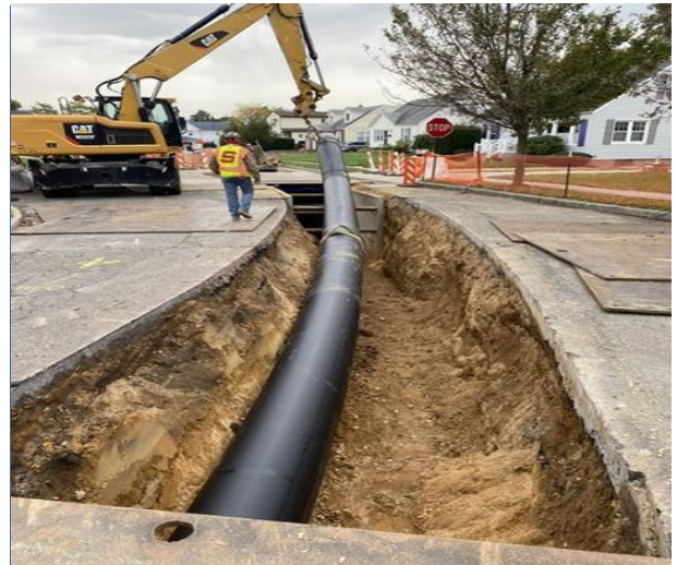
Installing HPDE Pipe in Trench on S Pershing Ave
