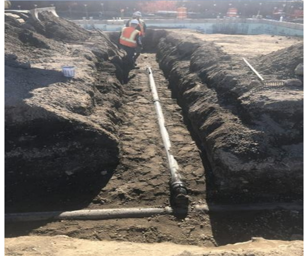
Installing Sanitary Sewer Piping Under Building Floor Slab
