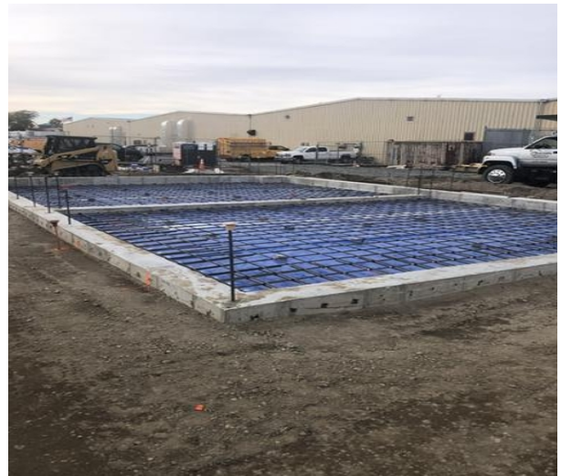
Rebar Installed for Chemical Rooms in Northwest Corner
