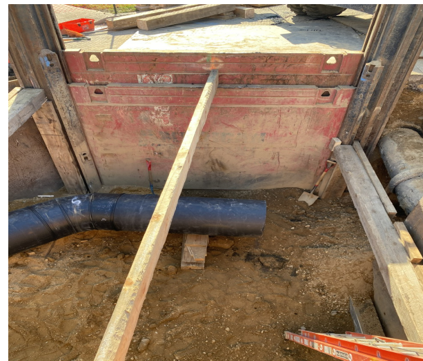
HDPE Pipe Fusion Pit on Brenner Ave
