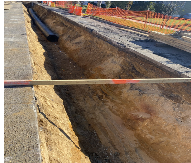
Installing HDPE Pipe on Brenner Ave
