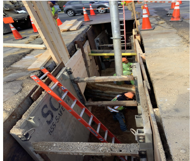
Installing Shoring for Trench Excavation on Central Ave
