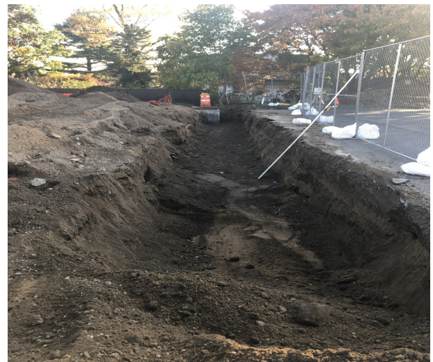
Compacting Sub-base for Retaining Wall on Site West Side
