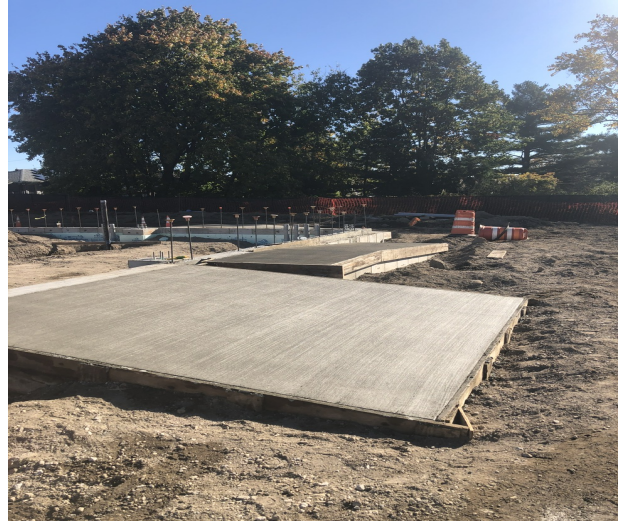
Concrete Ramps Installed on Building West Side
