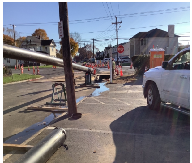
Inserting HDPE Pipe into Trench on Central Ave
