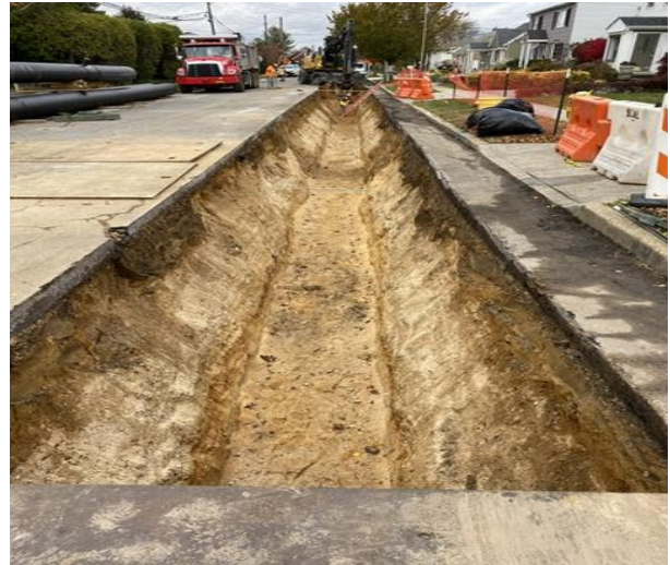
Excavated Trench on S Sheridan Ave
