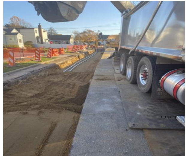
Backfilling Trench on S Sheridan Ave
