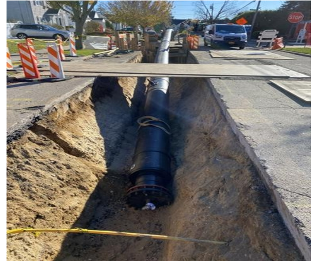
Installing HDPE Pipe on S Sheridan Ave
