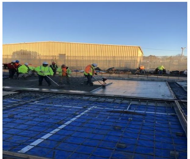
Finishing Concrete Floor Slab on Building North Side
