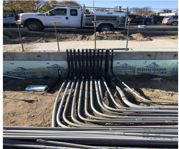
Conduits Installed in Building Electrical Room
