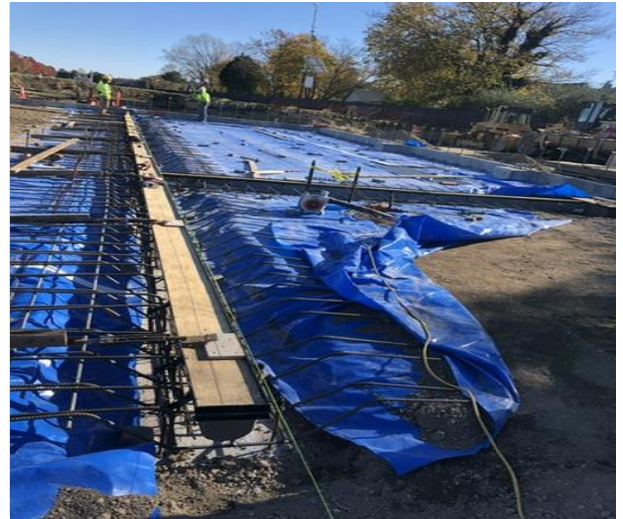
Installing Rebar for Building Southern Trench Drain
