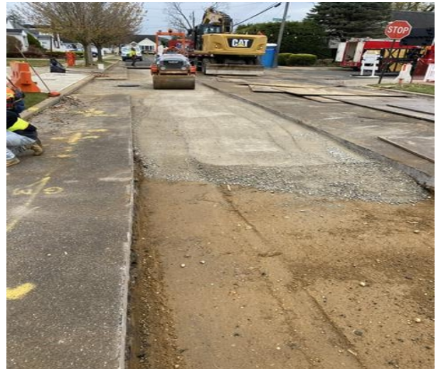
Backfilling Trench on S Sheridan Ave
