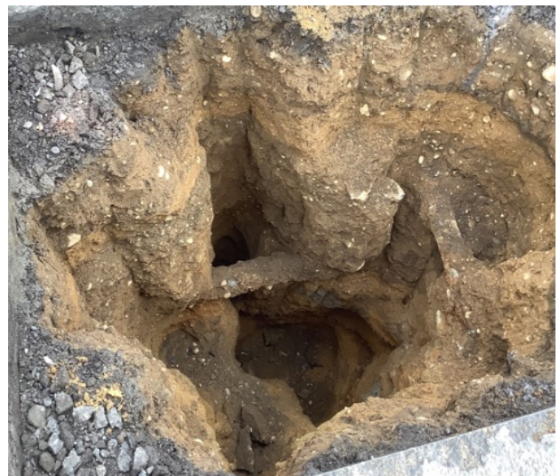
Conducting Utility Location on Central Ave Near Hickey Blvd
