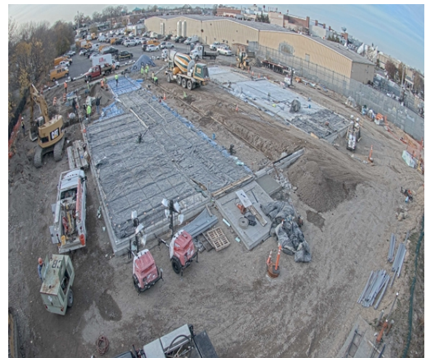
Aerial View from East Side of Site
