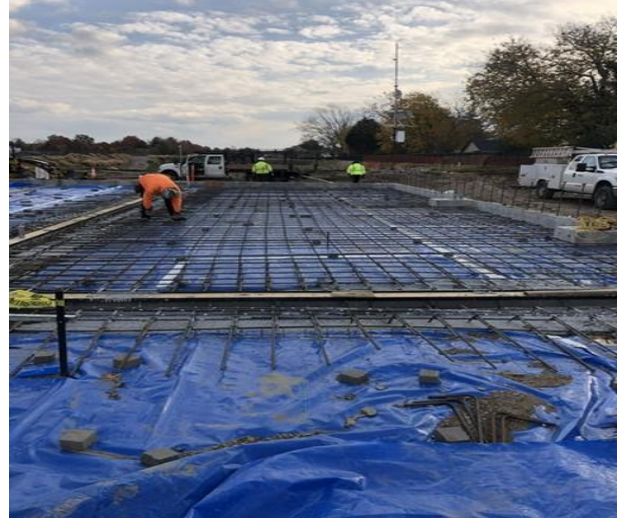
Installing Rebar for Floor Slab in Southeast Corner
