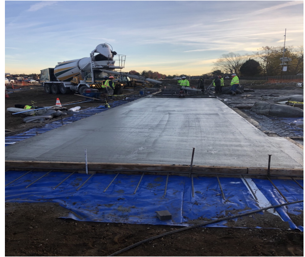
Finishing Concrete Floor Slab North of Southern Drain
