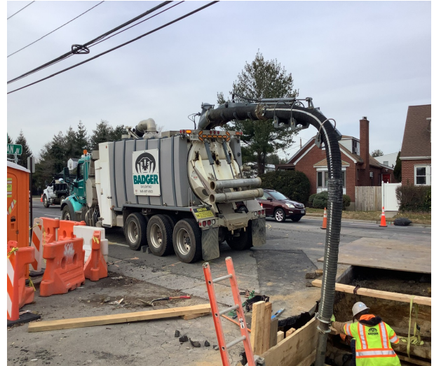
Excavating Trench With Vacuum Truck on Central Ave
