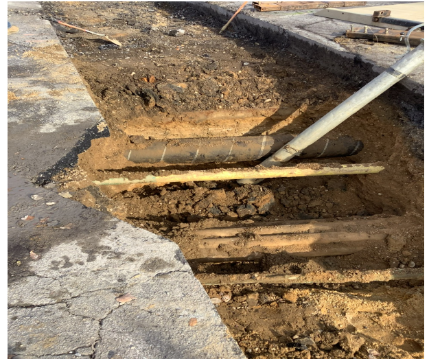
Numerous Utilities Located in Trench on Central Ave
