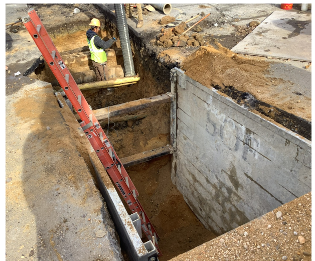
Installed Trench Box on Central Ave
